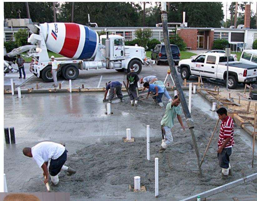
Left: Concrete slab was poured so that room floors slope to their respective central drains.
